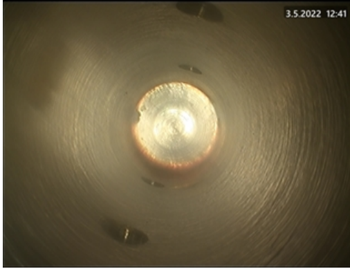
Burner #14_vane hole
